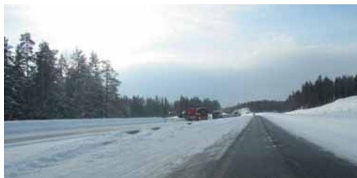
Figure 5.2 An over-ride incident in Sweden where the road median barrier has lost its function mainly due to the snow heaps
